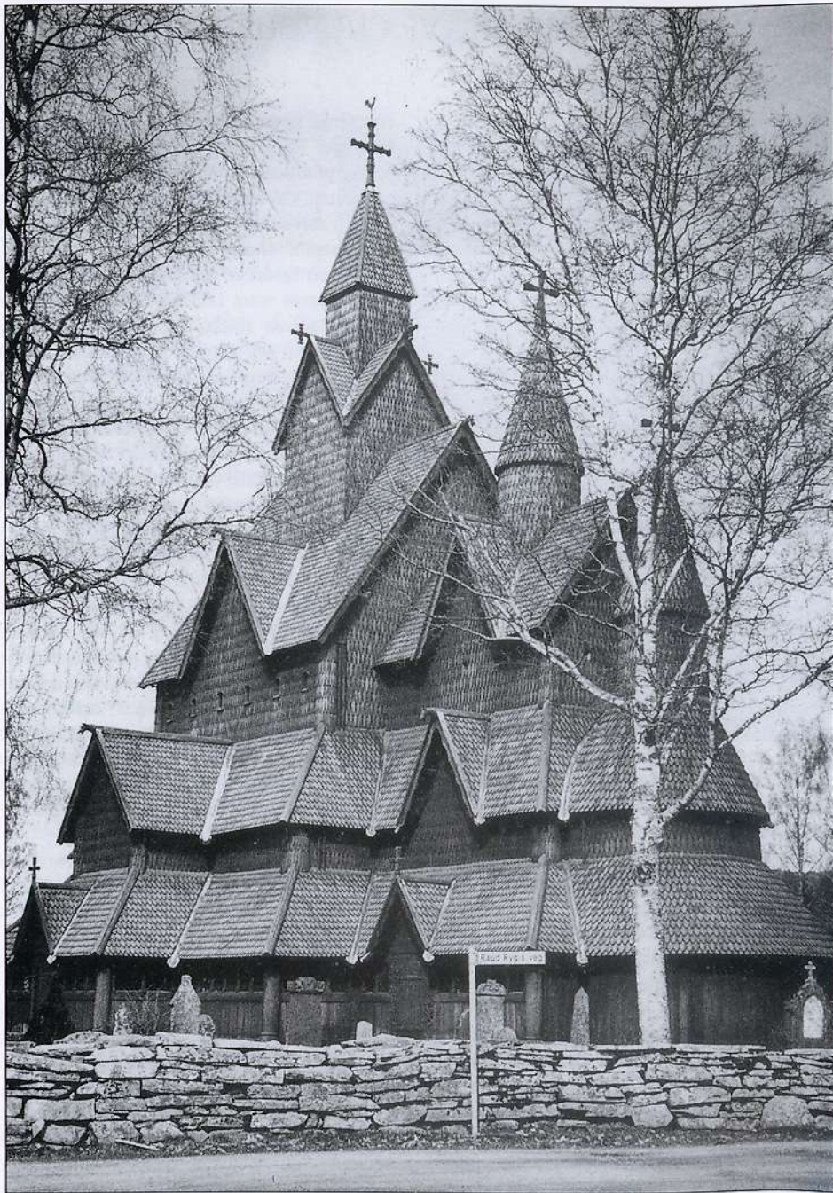
Heddall stave church is Norway's largest. Dedicated in 1147 and completed around 1250, it is triple-naved with an apse, and surrounded by a covered single-storey ambulatory. Its interior was extensively decorated with Telemark (Rose painting) in the 17th century. Kodochrome 64
