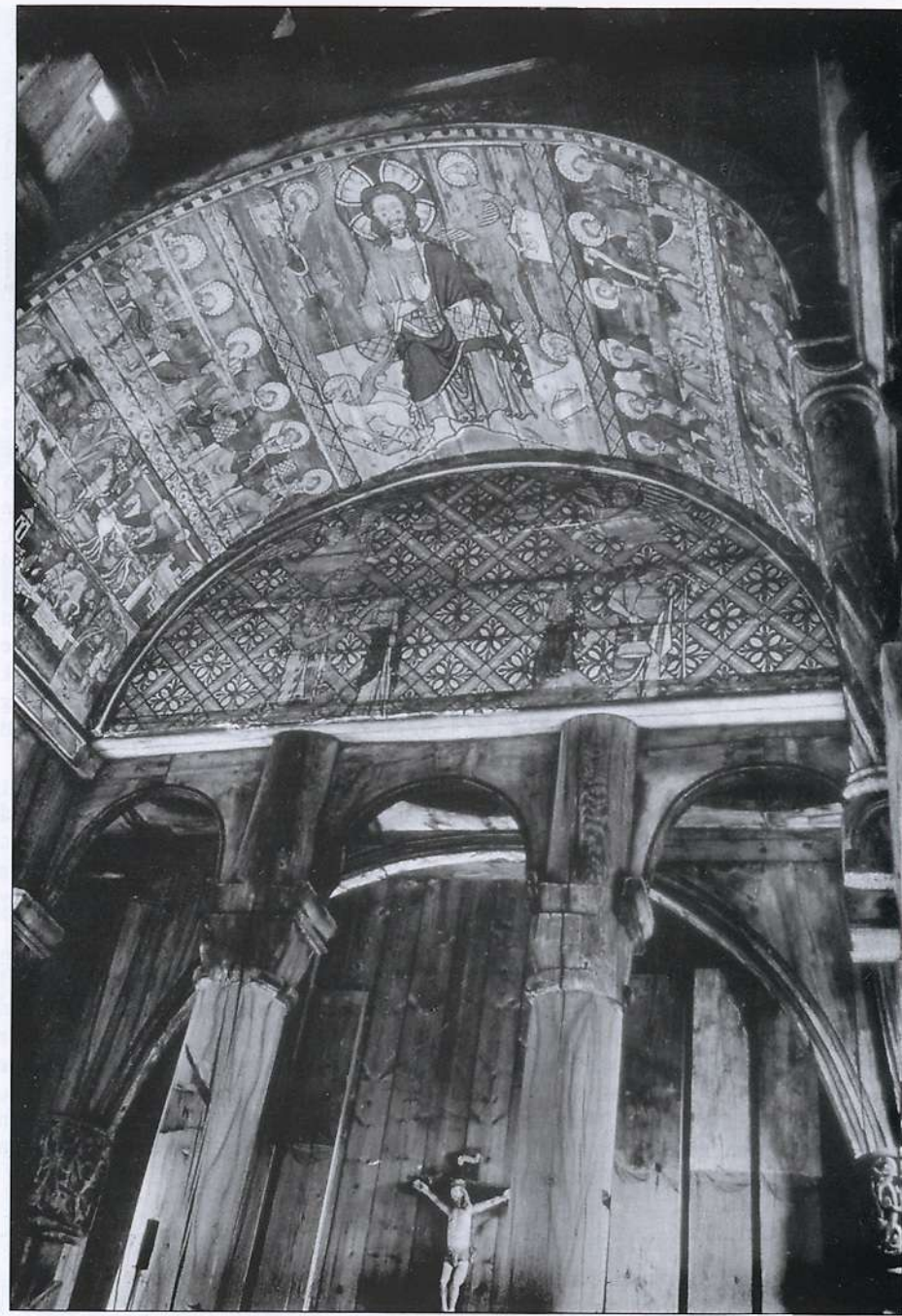
Torpo stave church, oldest remaining building in the Hallingdal, was dedicated to St Margaret in the late 1100s. Its ornate ceiling canopy was painted in the 13th century. The typical stave up-rights and ceiling framework are clearly evident. (Kodachrome 64, 8 seconds at f5.6)
